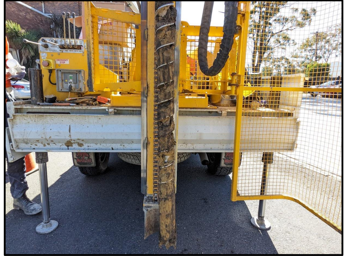
Figure 13. Drilling of BH8.
