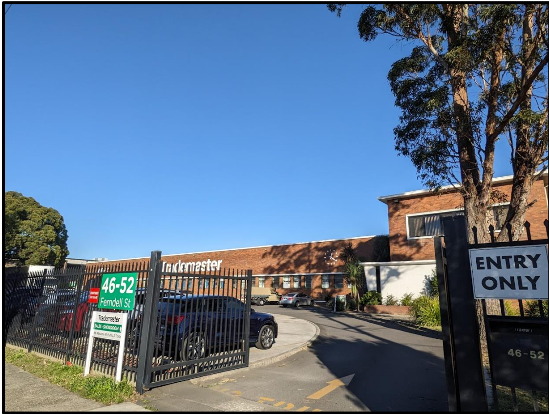
Figure 8. Entrance gate to the site.
